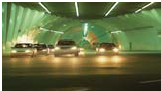
LED tunnel light single lamp intelligent upgrading project at the Yan'an Tunnel in Shanghai
