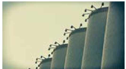
Intelligent industrial lighting control system in Philippines
