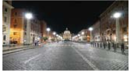
Intelligent LED single street lamp control project in Italy
